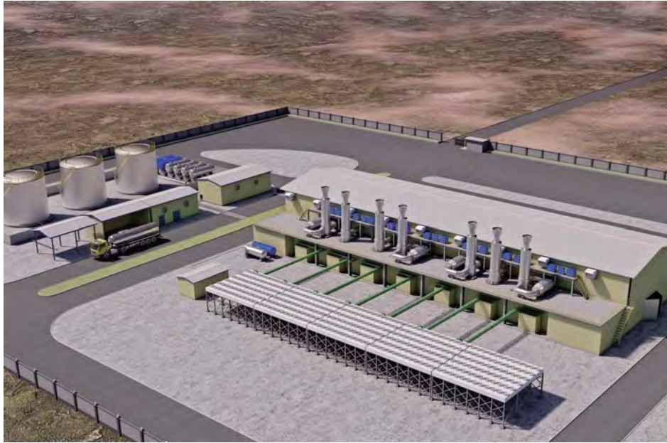
MAN 12V32/40 40MW, 11KV, 50HZ, Captive Power Plant
