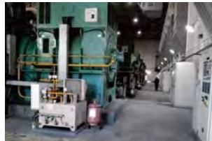
33MW, 13.8KV, 60HZ, Base Load, to the National Grid
